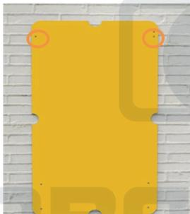
1. Use the positioning cardboard (provided in accessory package) and mark the screw hole positions on the wall, as shown in the four holes on the left.
