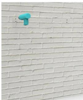
3. Press the marked position with the electric drill and trepanning 4 holes with a diameter of 10mm on the wall. The hole depth shall be greater than 70mm for fitting the expansion bolt of M6.
